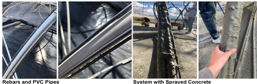
Figure 3. System Implementation with Concrete
