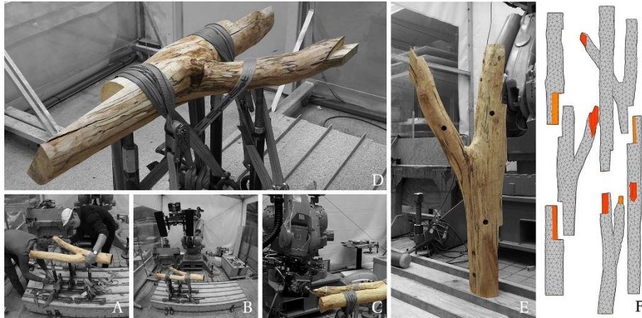
Figure 4: Workflow: a) mounting, b) scan, c) cut, d) demounting, and e) machined forked, and f) individual element with joinery geometry.
